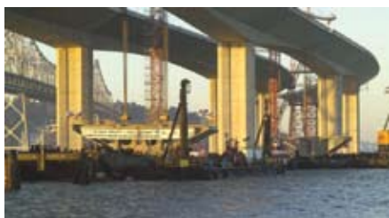
Fig. 4: The San Francisco-Oakland Bay Bridge Skyway
