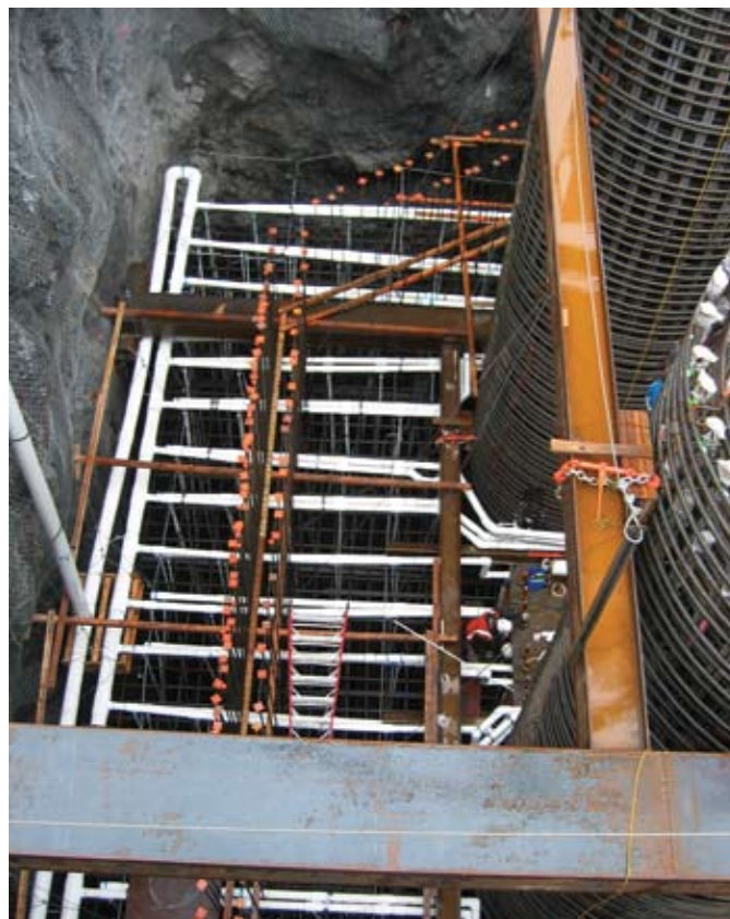
Fig. 6: PVC cooling pipe system for one of the footings supporting a pier for the San Francisco-Oakland Bay Bridge
